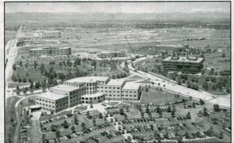
The Class A building at 9800 S. Meridian Blvd. is one of the most prominent buildings in the southeast market.
